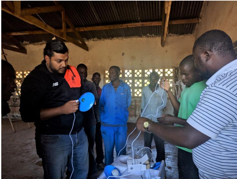
Installation of a solar system at Kakoma Primary School
